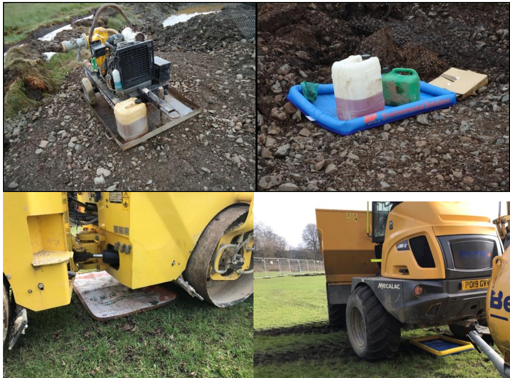
Plate 2: examples of dip pan, bunds and EnviroPad
